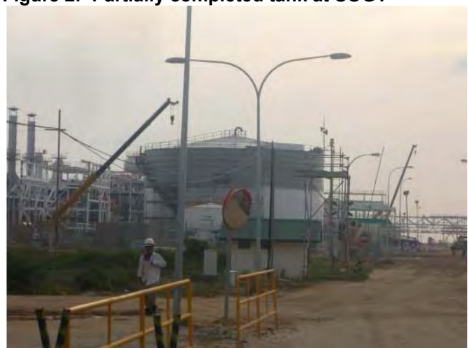
Figure 2: Partially completed tank at SOGT
