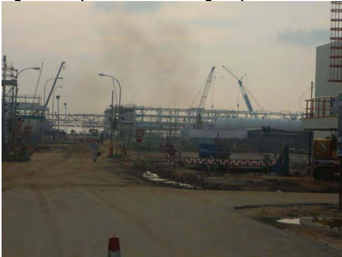
Figure 3: Superstructures taking shape
