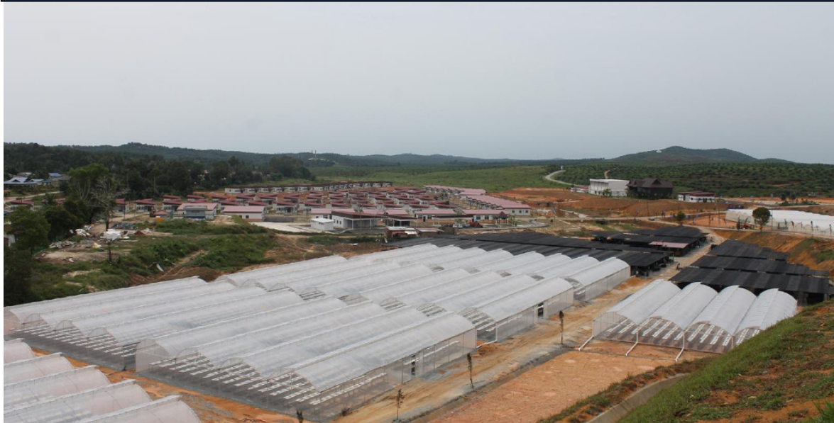
Figure 4: 1 st completed Sentuhan Kasih project in Tenggara, Johor
