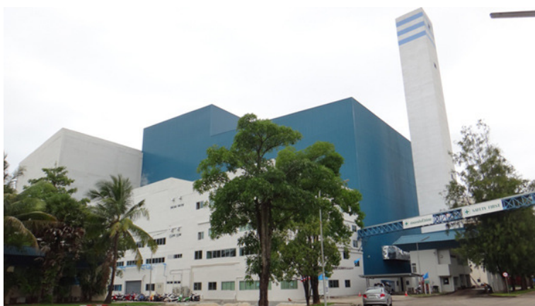
Figure 5 : Phuket Municipal Solid Waste Incineration Power Plant
